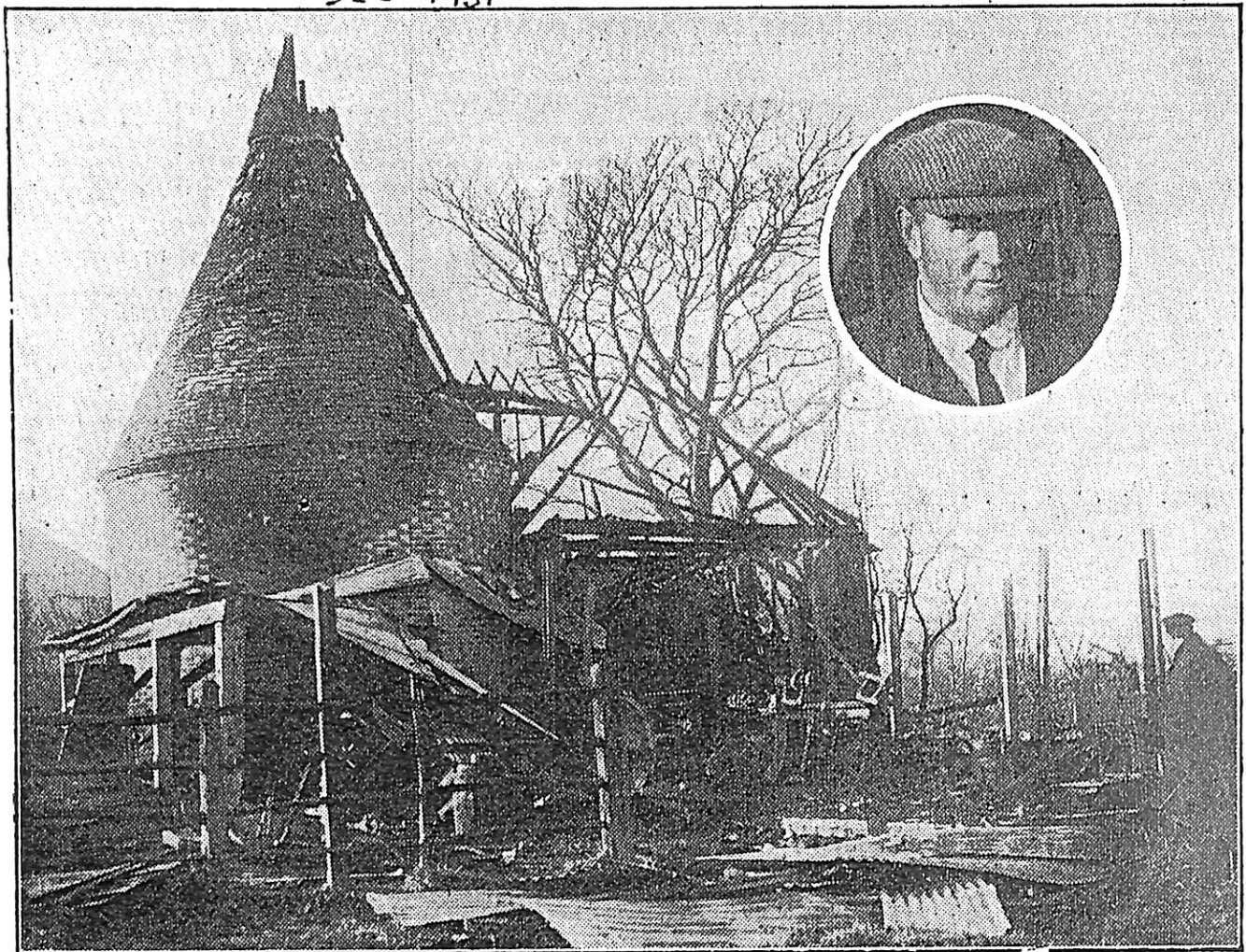
THE RUINS CAUSED BY THE DISASTROUS FIRE AT OLD SURRENDEN, BETHERSDEN, ON SUNDAY. INSET:—MR. T. BATT, THE OCCUPIER OF THE PREMISES, PART OF WHICH WAS USED BY HIM FOR THE REPAIR OF MOTORS AND MACHINERY.
